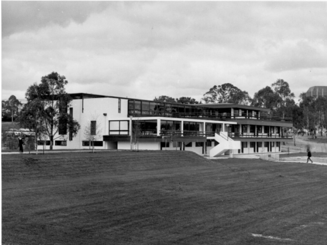
Figure 3. Newly completed union building, October 5 th 1965. (Source: Godden Mackay Logan, ANU Heritage Study Acton Campus Volume 2: Heritage Inventory , prepared for the Australian National University, August 2012, p.95 - ANU Archives)
